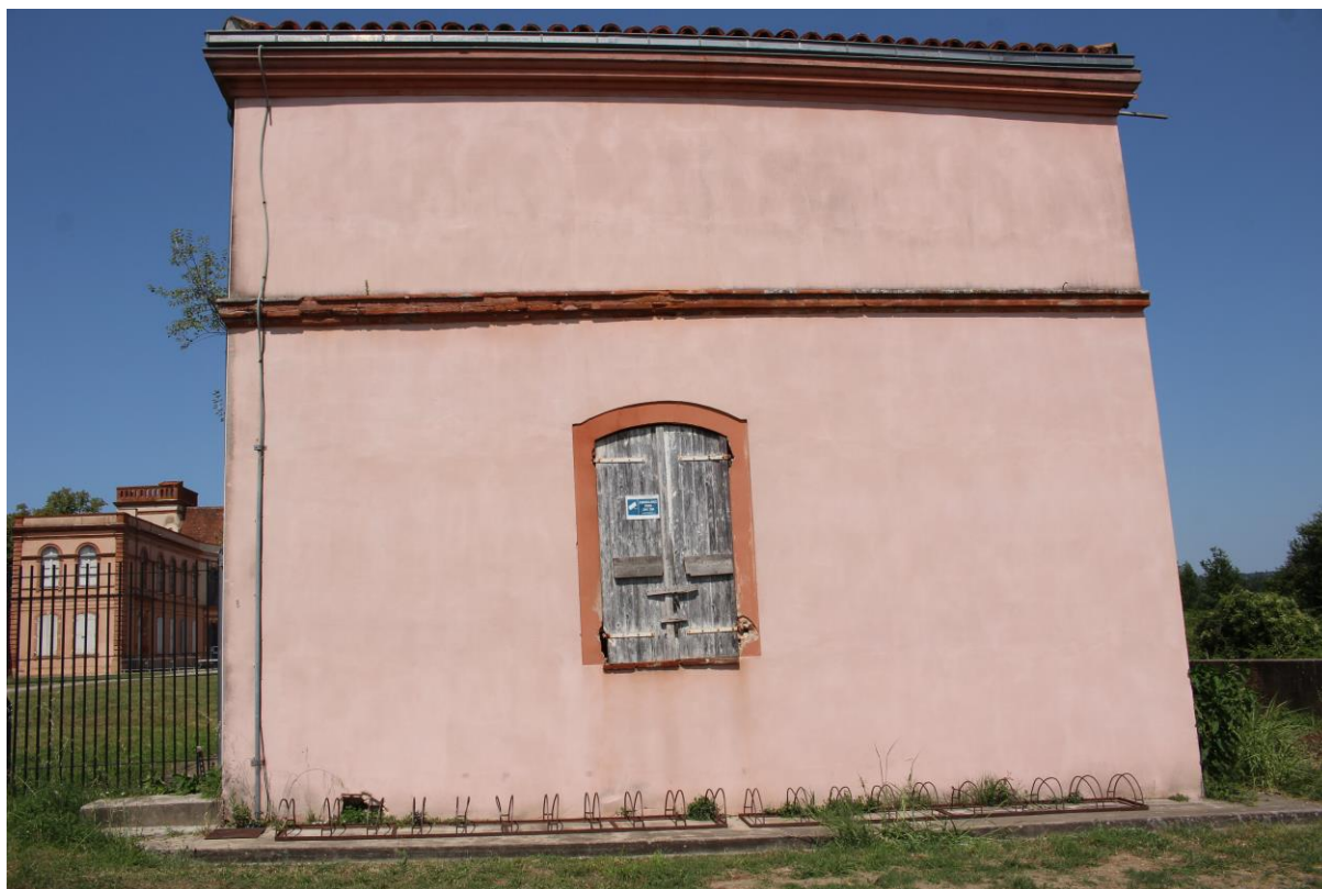
Fig.19 – VUE DE LA FACADE SUD – BATIMENT 3, ENSEMBLE ARIEGE
