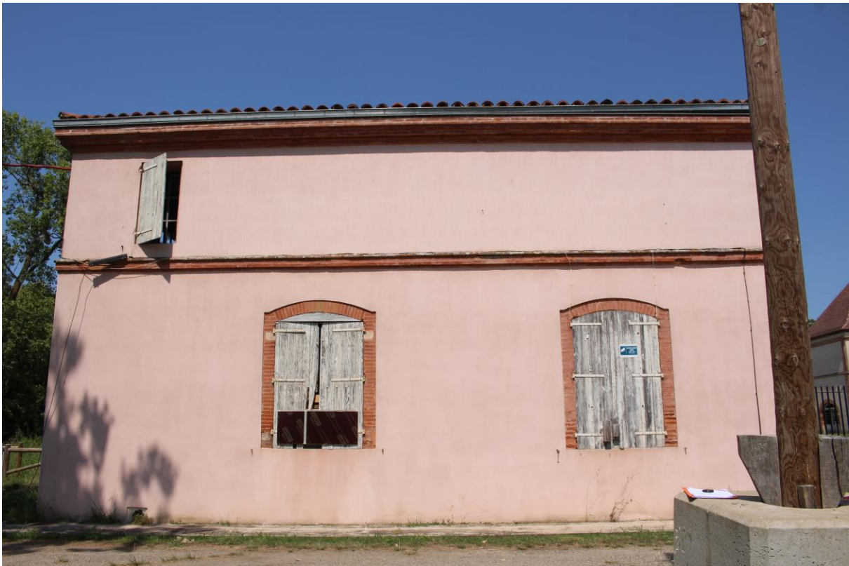
Fig.16 – VUE DE LA FACADE SUD – BATIMENT 2, ENSEMBLE GARONNE
